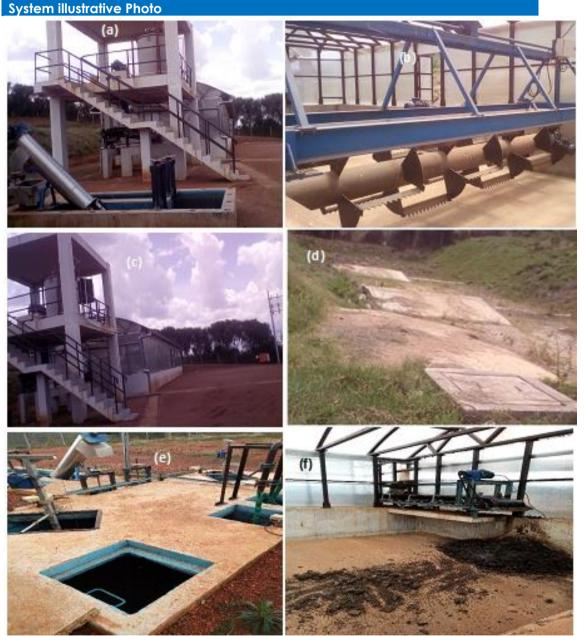
Figure 46: Components of Faecal sludge treatment systems for Nyagatare, Kayonza, Nyanza and Gicumbi landfills including grit removal (a), Screw press for thickening sludge(b), Green house for solar drying bed (c), infiltration pit for wastewater (d), Waste water treatment chamber (e), Treated and stabilized Sludge (f).
