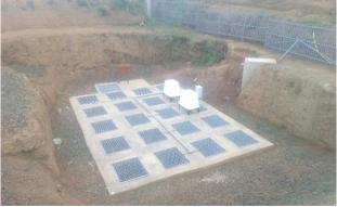
Figure 32: Septic Tank for wastewater pretreatment at UR Nyarugenge
