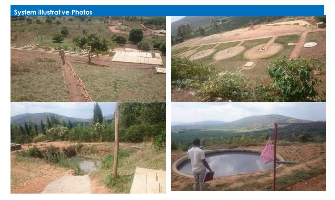
Figure 35: Components of Mageragere sewage treatment system: Constructed wetland (a), Series of Biogaz Digestor tank(b), effluent receiving pit before to be discharged into environment (c) and Influent receiving tank (d)
