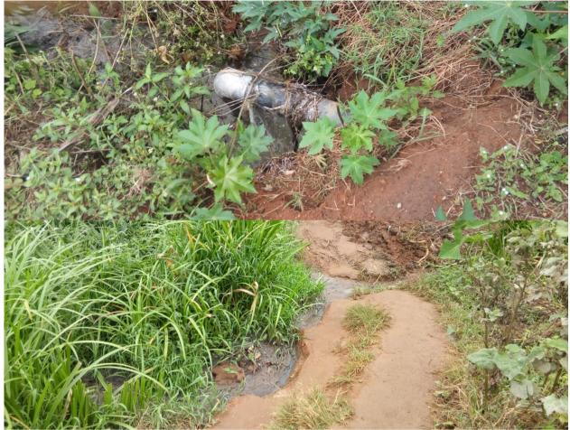
Figure 30: Juru estate Fresh faecal material discharge to open environment
