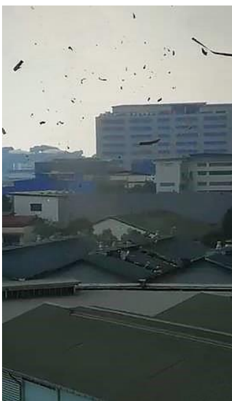
Figure 8: A landspout ripped off parts of a factory building's roof at Gul Way in the Tuas area (Source: STOMP)
